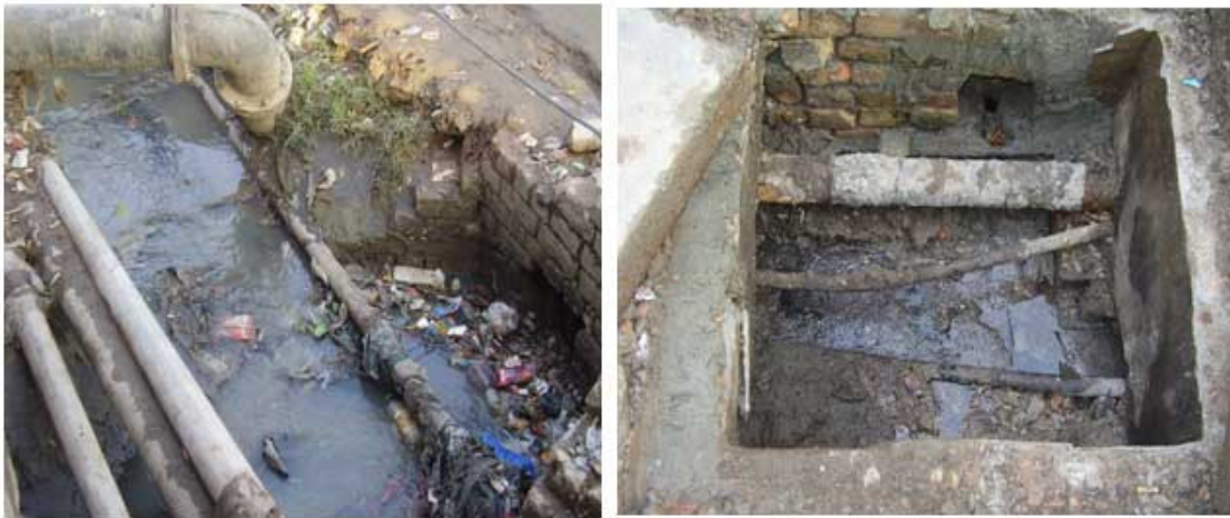
Fig. 8.1: Hand in gloves laying of drinking water distribution pipe lines with sewerage drains.
